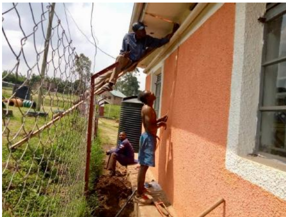
Installing Lightening Arrestors on a Classroom
